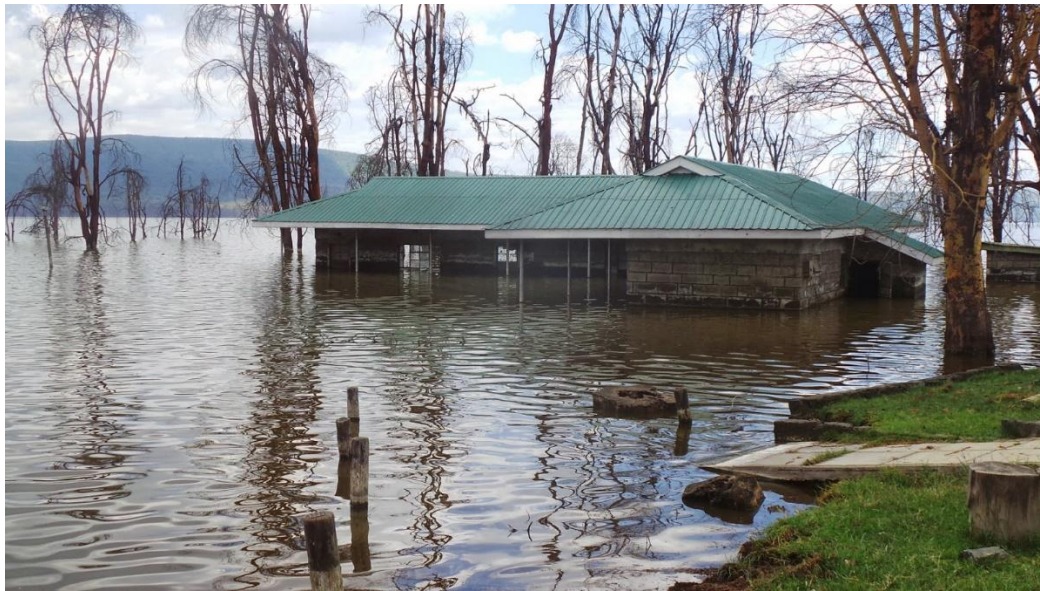
Figure 1: Impacts of fluctuating lake water levels on infrastructure at Lake Nakuru National Park
