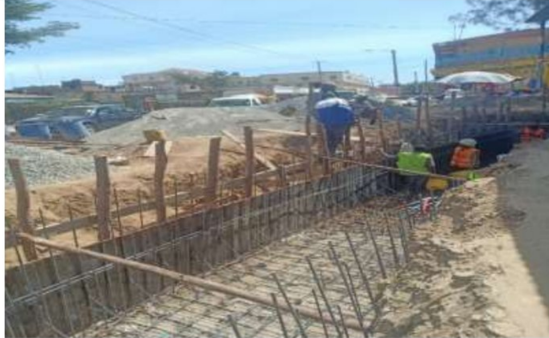
Box culvert Drainage along Mama Ngina Street
